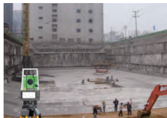
Foundation pit engineering
